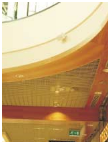
Shopping Center Jumbo, Vantaa, Finland, Elam wall and ceiling panels in cherry.
