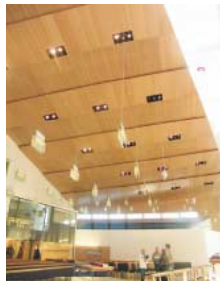
New church of Klaukkala, Finland, Elam wall and ceiling panels in oak.
