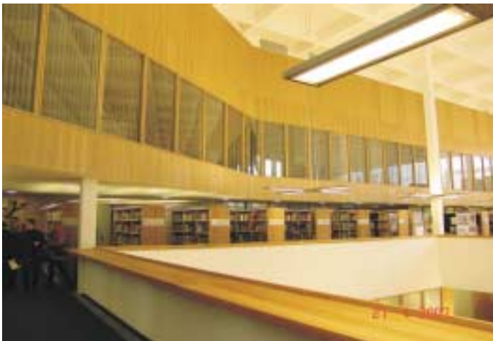
New Library of Turku, Finland, wall panels in waxed birch.
